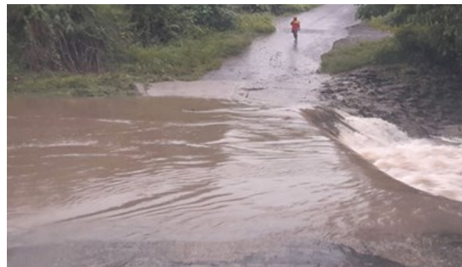
Figure 12d: Navula bridge, Saru, Lautoka on the 15 th . Source: Fiji Roads Authority.
