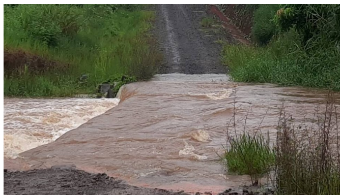
Figure 12e: Naqumu Crossing, Seaqaqa on the 15 th . Source: Fiji Roads Authority.
