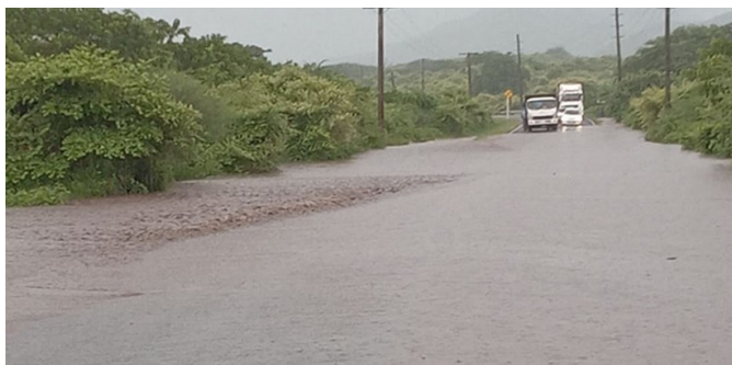
Figure 12a: Kings Road near Waisai Bridge on the 13 th . Source: Fiji Roads Authority.
