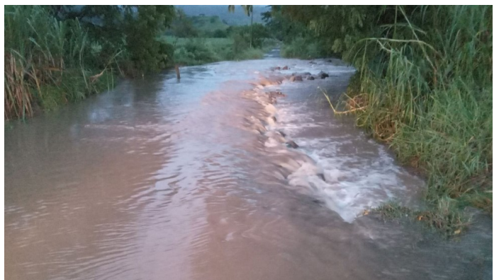
Figure 12n: Matacawa Road, Tavua. on the 19 th . Source: Fiji Roads Authority.
